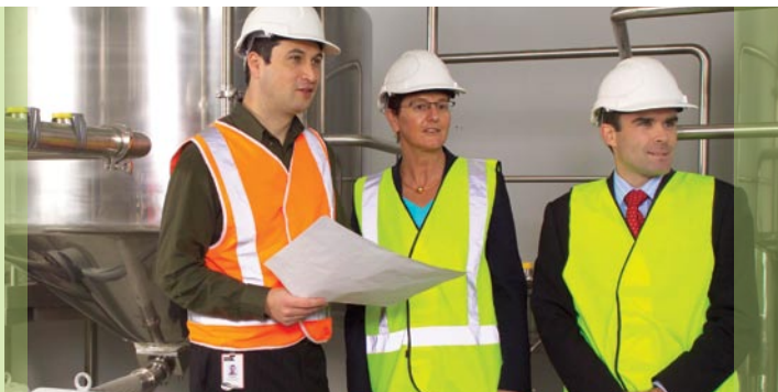
In Melbourne, construction of new influenza vaccine production facilities is on track to deliver CSL additional capacity in 2008. Checking progress in the ultrafiltration plant are Andrew Bervanakis, (Senior Project Manager, CSL Biotherapies), Mary Sontrop, (General Manager, CSL Biotherapies, Australia and New Zealand), and Cameron Barrett, (CSL's Director, IT and Facilities).
