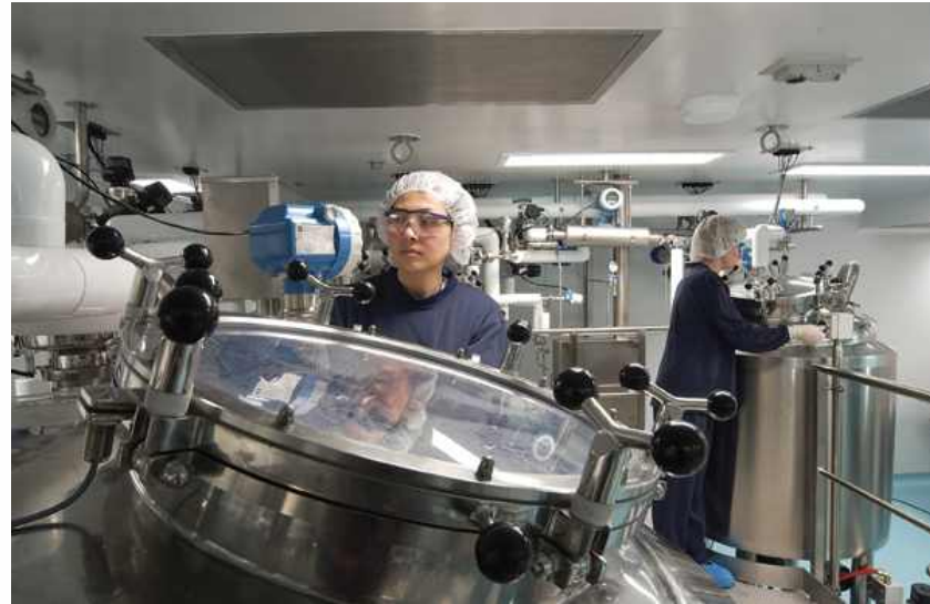
Buffer preparation area in CSL's new state-of-the-art influenza vaccine centre
