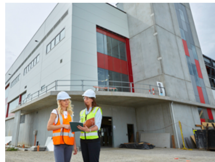
CSL Behring's new albumin production facility in Broadmeadows, Australia, is anticipated to receive regulatory approval in 2019.
