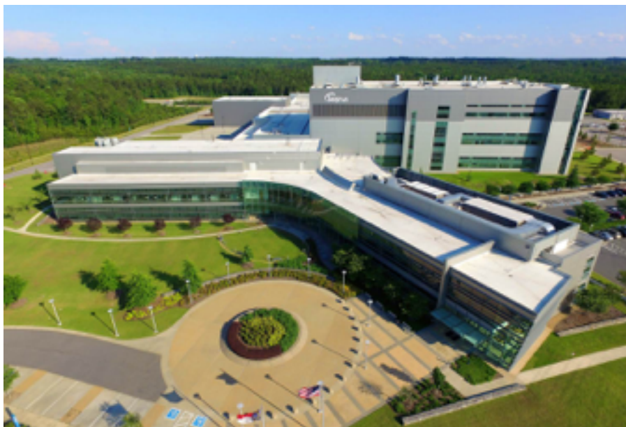
Seqirus' state-of-the art Holly Springs manufacturing facility in North Carolina, US. In an industry first, Seqirus has successfully produced cell-based influenza vaccine at commercial scale using a candidate vaccine virus that has been isolated and grown in cells, rather than in hens' eggs.
